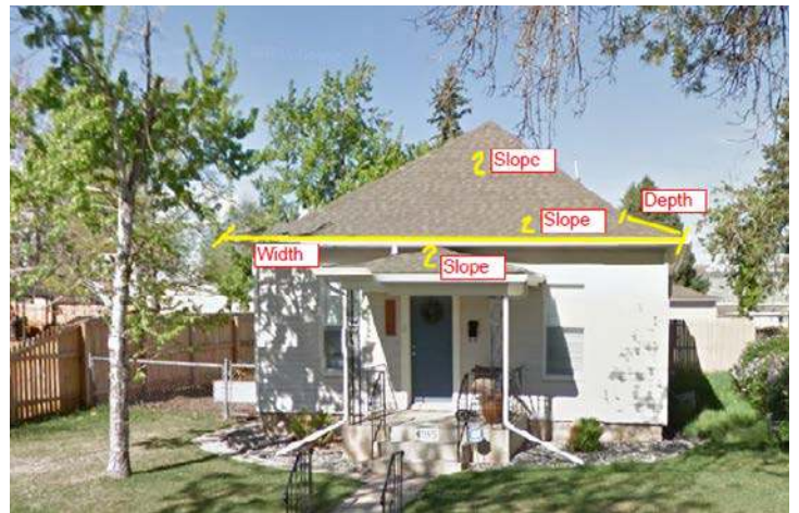
Figure 2: Roof that resulted in inaccurate measurement
